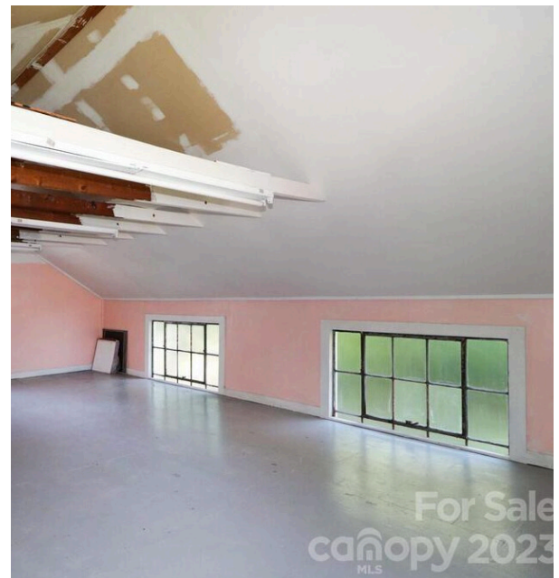
Inside shot of garage showing how the windows looked in bonus room before being covered up
